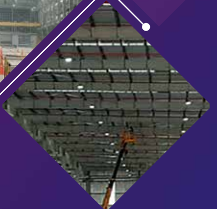
Warehouse at Lucknow
